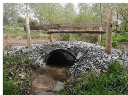
Exemple de franchissement type hydrotube (Agev solutions)
