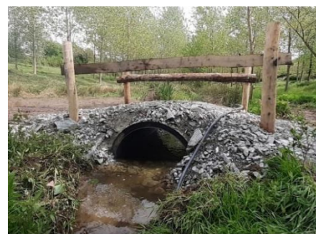
Exemple de franchissement type hydrotube (Agev solutions)
